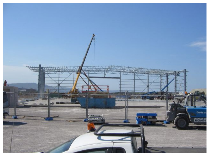
The framework structure well advanced last week
